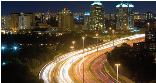
Figure 1 – High mast streetlights along a highway in Canada.
